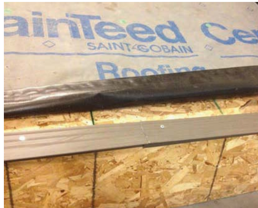
4. After the drip edge is completely installed on eaves, install MetaLayment/WinterGuard® over the drip edge in accordance to local building codes, followed by DiamondDeck®.
