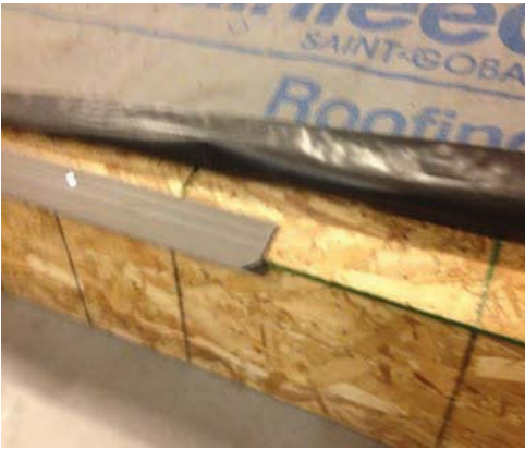
1. Cut and bend drip edge trim on the outside to conform to rake edge and inner and outer gable.
